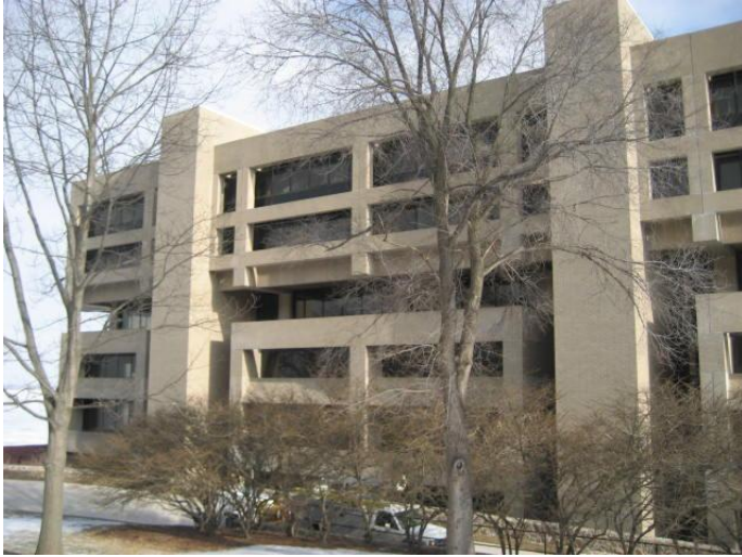
Picture #13: West Elevation Office Tower looking Northeast
