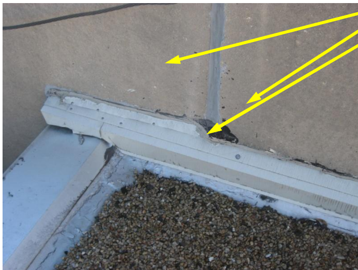
Picture #17: Flashing behind misaligned panel
