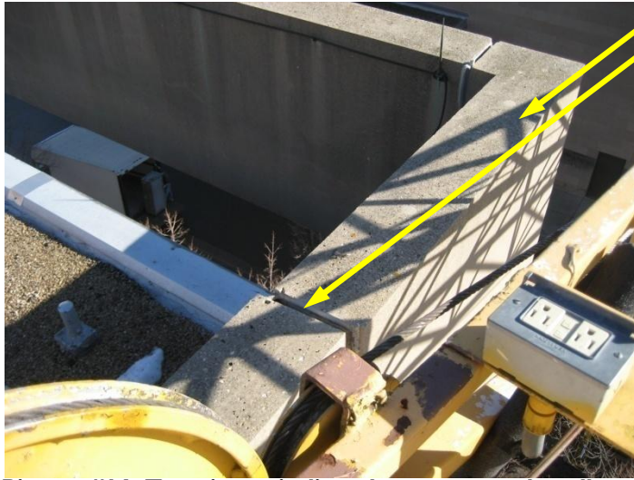
Picture #16: Top view misaligned parapet-south wall
