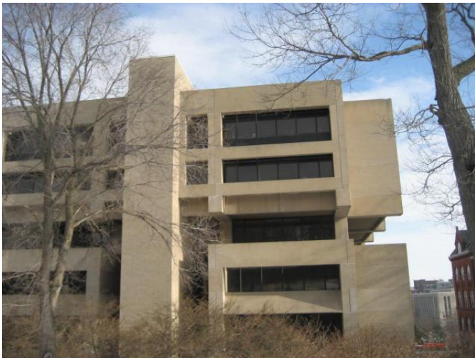
Picture #14: West Elevation South End
