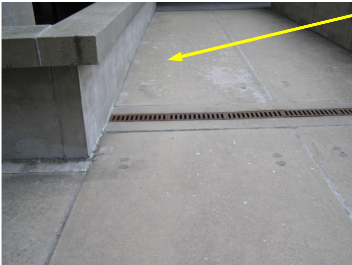
Picture #30: Center Section of Walkway showing spalled panel
