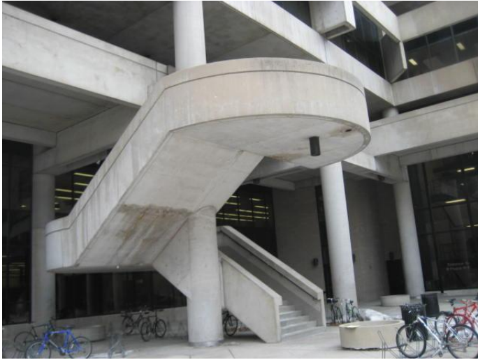
Picture #23: Concrete Stair at Main Entry Plaza
