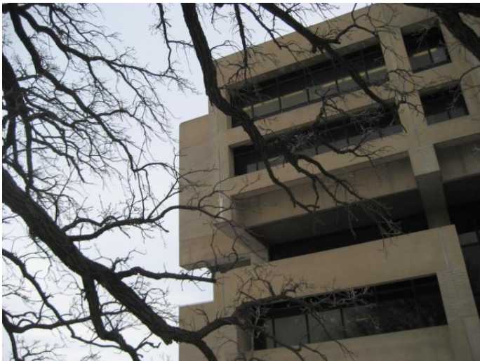
Picture #12: West Elevation Office Tower North End
